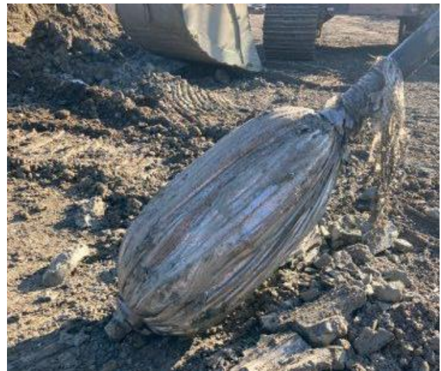
Figure 12. Exhumed EB anchor
